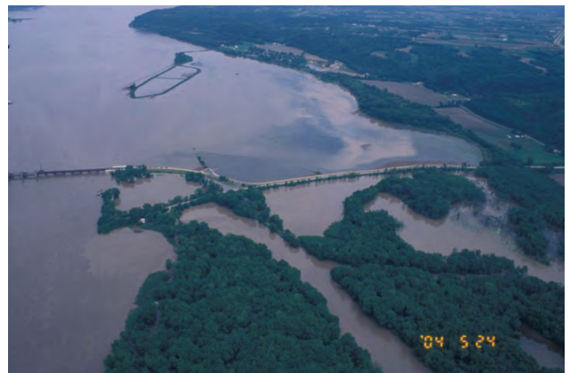
Photo 10. Downstream of Site Looking North
