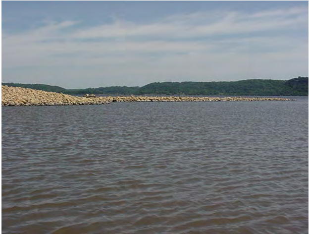
Photo 22. Rock Spur Dike
