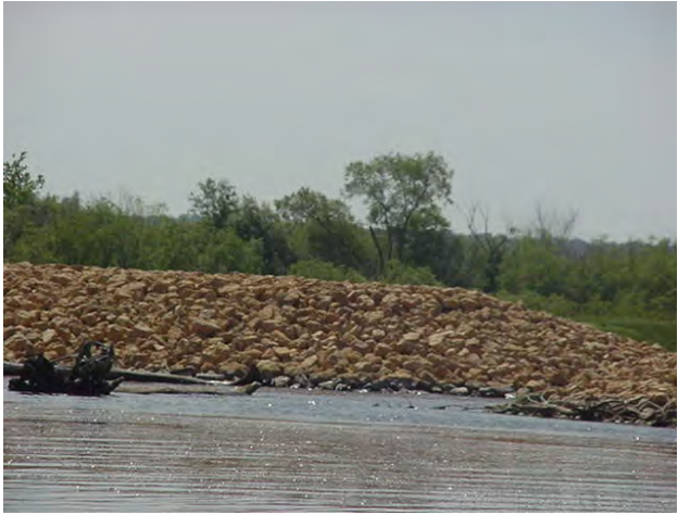
Photo 16. Erosion Protection on Embankment B
