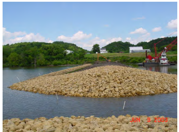
Photo 5. Flow Inlet Structure
