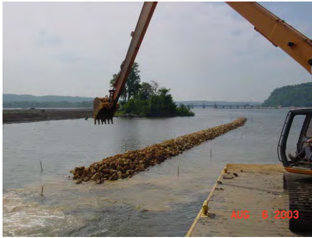
Photo 12. Construction of Riprap Dike
