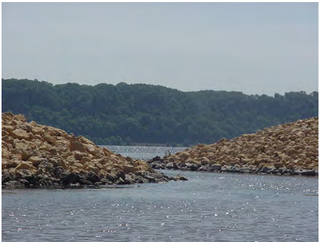
Photo 18. Flow Inlet Structure
