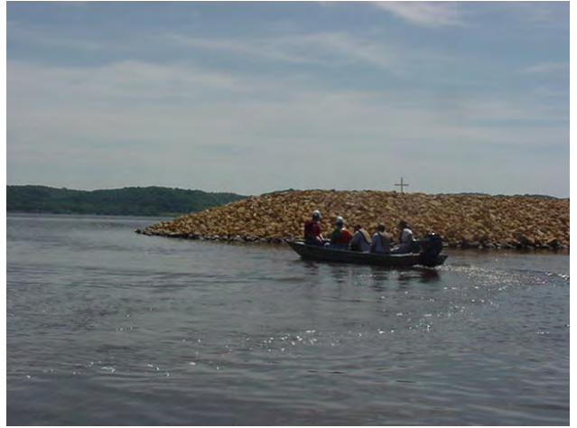
Photo 19. Erosion Protection Embankment B
