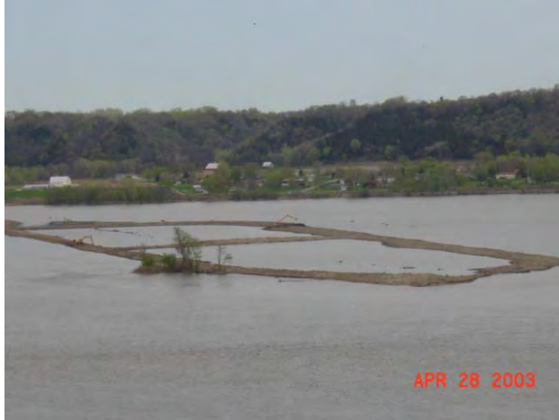
Photo 11. Island and Confined Disposal Facility Construction
